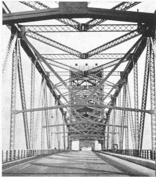
MARINE PARKWAY BRIDGE, SHOWING OPEN TYPE OF FLOORING.
